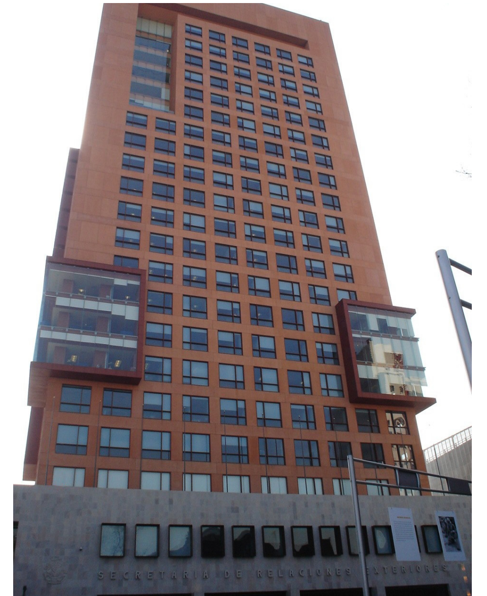
Figure 1. The office building of Mexico's Secretario de Relaciones Exteriores (Secretariat of Foreign Affairs).
